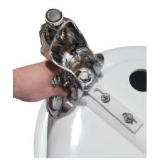
5. Before fully tightening the clawfeet to the brackets with a 19mm socket, double check how the face of the clawfoot lays on the tub and make adjustments if needed.
